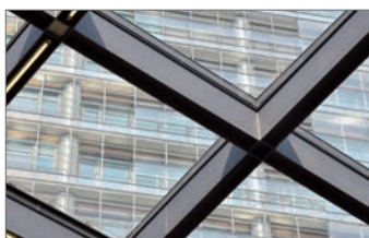
METALLBAU METAL CONSTRUCTION
