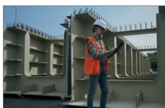
STAHLBAU STEEL CONSTRUCTION
